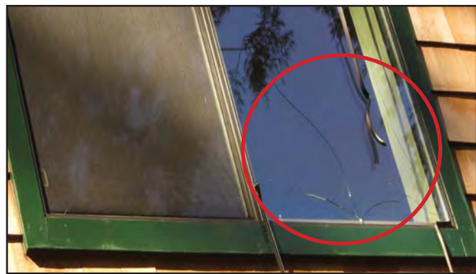
A structure fire at the arrow burned into nearby trees. Radiant heat cracked the window shown in the red circles.
