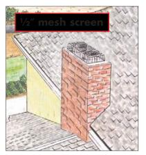
Burning embers landing on wood shake roofs are one of the leading factors for losing your home to a wildfire. Replace your wood shake roof with non-flammable (Class-A) roofing materials such as asphalt shingles, tile, or metal.
