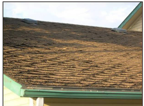
Though it may have originally had a Class A rating, this old, weathered asphalt composition shingle roof would no longer provide adequate protection against embers and heat.
