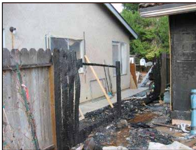
Create non-combustible space between the wood fence and the house walls with metal gates, and similar material.
