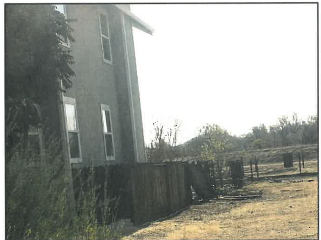
Create non-combustible space between the wood fence and the house walls with metal gates, and similar material. This fence would have burned to the house walls had firefighters not arrived to extinguish the fire.
