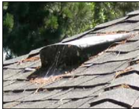
Through-roof vent
