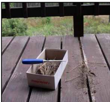
Keep needles and debris from accumulating between deck boards or between deck and siding.
