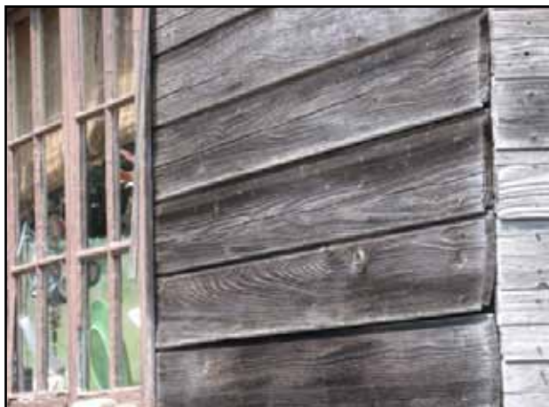
Home on left is vulnerable to wildfire because of its aging, shrinking wood siding and single pane windows. Home on right was retrofitted with fire-resistant siding, boxed eaves, metal-clad fascia and double-paned windows.
